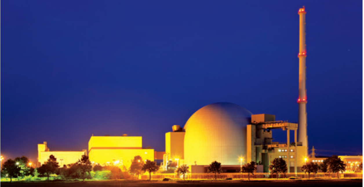
Nuclear power station
